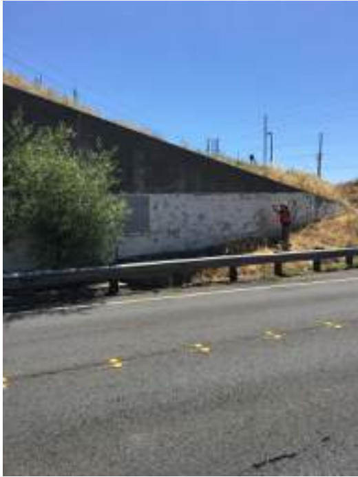
Photo 4 – Eastern abutment, southern face, viewed east.
