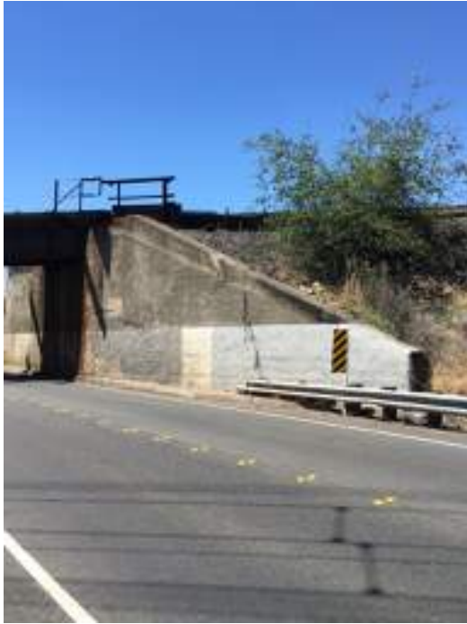
Photo 2 – Western abutment, northern face, viewed west.
