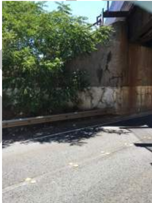
Photo 3 – Eastern abutment, northern face, viewed south.
