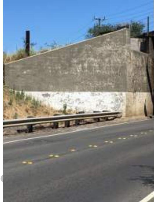
Photo 1 – Western abutment, southern face, viewed north. 12/20/16
